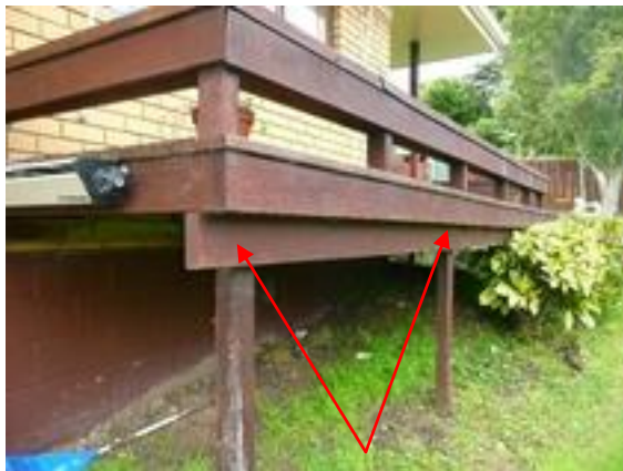
Intended location of new bolts (2)
