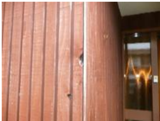
Fill holes, corner gap & re-stain
