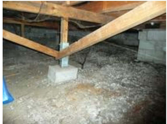
Brace pile & block perimeter footing
