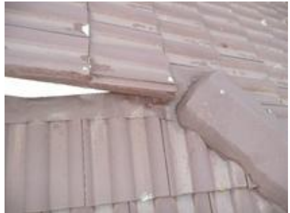
Well designed & installed lead flashings
