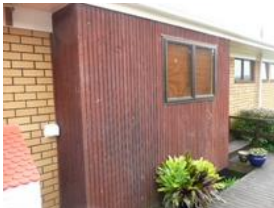
Recently painted fascia and eaves
