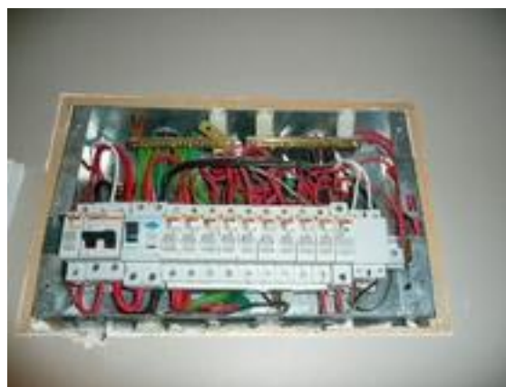
Standard miniature circuit breakers
